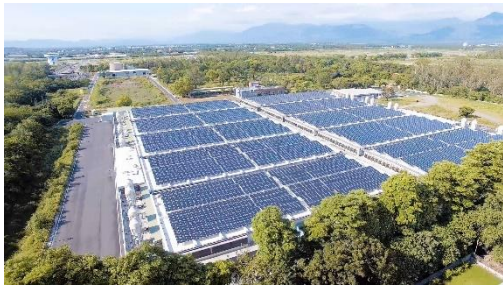
台糖東海豐豬舍屋頂型太陽光電 TSC DHF agricultural circulation pig farm roof-mounted solar panels
